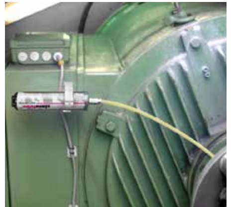
With the simalube 250ml lubricator, the generator is continuously supplied with lubricant for up to 12 months.
