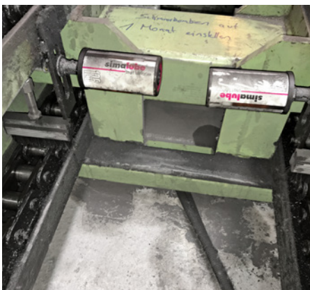
simalube lubricators, including brushes, are installed on a chain conveyor. The chains are thus continuously lubricated while being cleaned at the same time.
